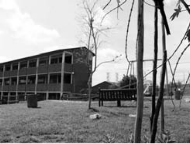
Photo 14. School Built as Part of the Alexandra Renewal Programme
