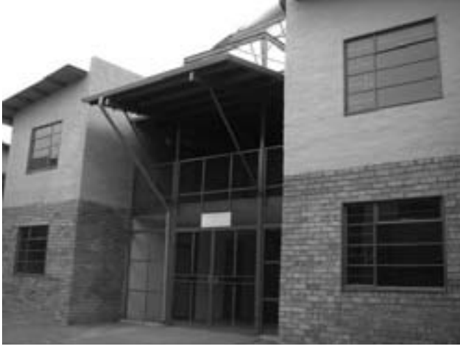
Photo 10. Housing Managed by JOSHCO in Alexandra
