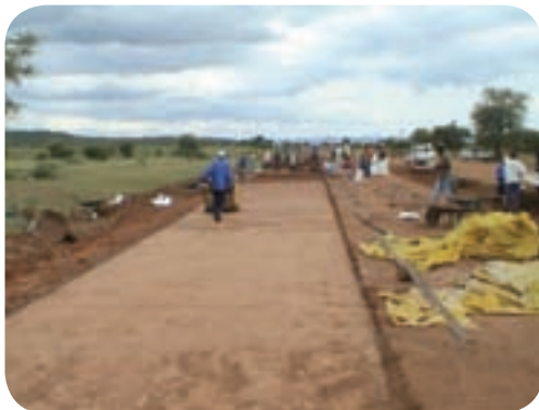
Compacting with walk-behind roller
