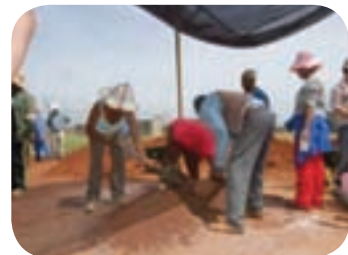
Mixing soil and stabilizer and adding water
