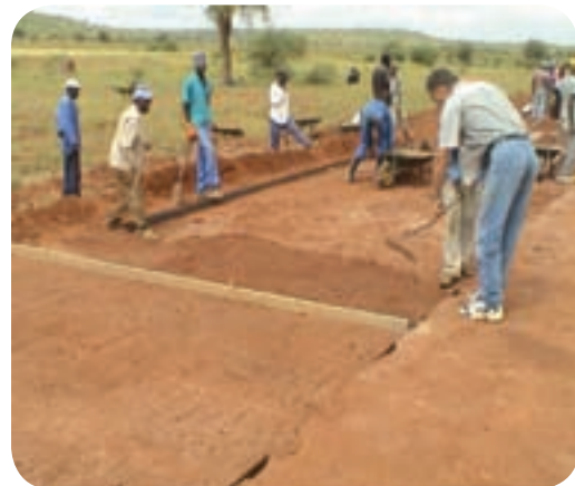
Shaping the stabilized layer
