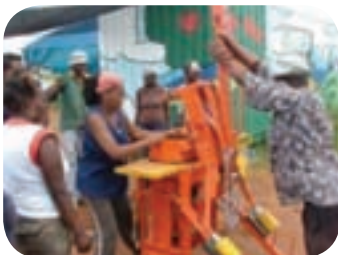
Pressing the earth blocks
