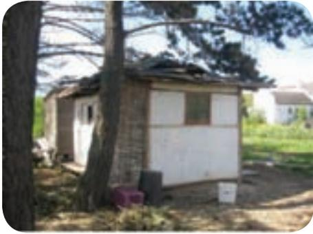
This little gum, wattle and hemp house was built at Ouden Molen, in Pinelands, Cape Town. It has a gum pole frame with an interlocking wattle basket weave (both invasive aliens), filled in and plastered with locally sourced clay and painted with lime.
