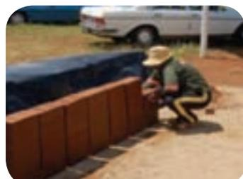
Stacking blocks for humid curing
