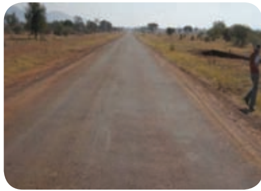
The Otta seal-surfaced road, still in good condition three years later
