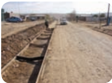
Constructing the side-drain next to the stabilized road
