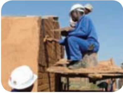
Plastering with local earth plaster (natural colour of local soil)
