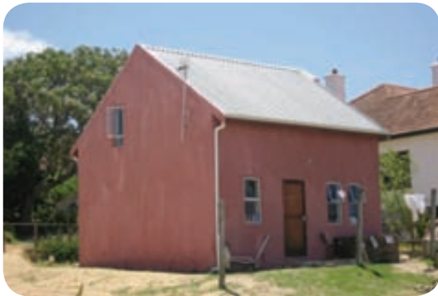
Hydraform brick house, Lynedoch Ecovillage, Stellenbosch
