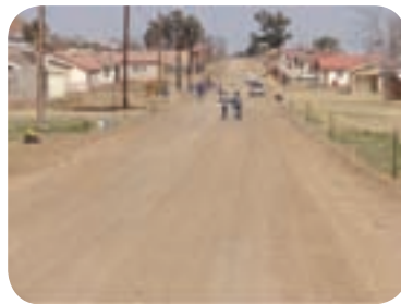
The road after stabilization and compaction, providing a safe, all-weather driving
