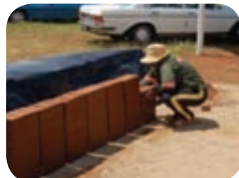
Stacking blocks for humid curing
