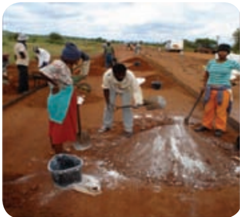
Mixing the stabilizer with the in situ soil
