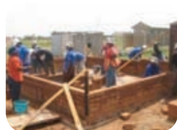
Training on building with CSEBs and local earth mortar
