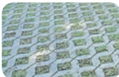
Examples of permeable paving
